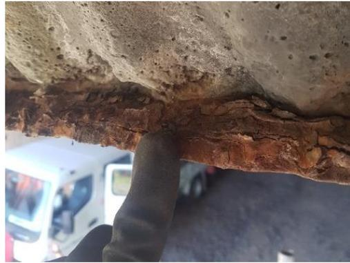
**Figure 9:** Typical section loss.
