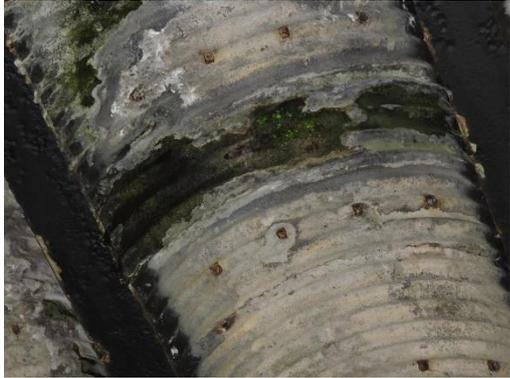
**Figure 7:** Typical example of water leaks through the deck.
