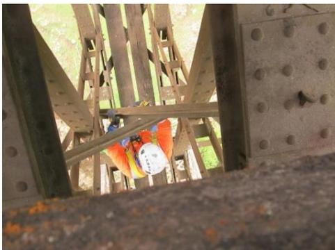
**Figure 3:** A qualified coating inspector in action.
